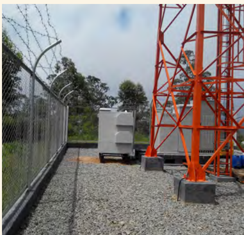
Figure B4.1.1 Methanol fuel cells in Indonesia's telecommunications sector
