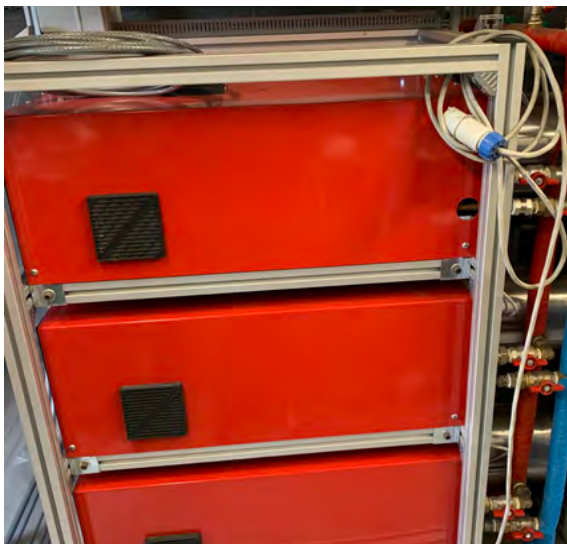
FIGURE 4.3 Hydrogen boilers deployed at Shapinsey School, Kirkwall, United Kingdom
