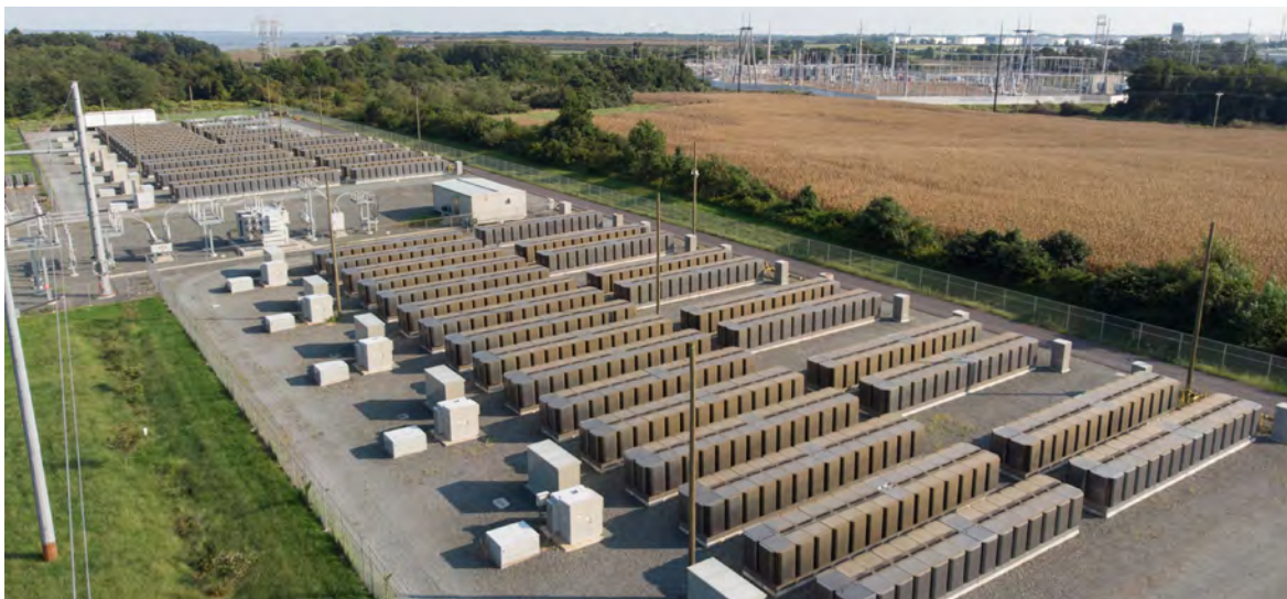
FIGURE 4.5 Utility-scale fuel cell solutions: Solid oxide fuel cell units in the US
