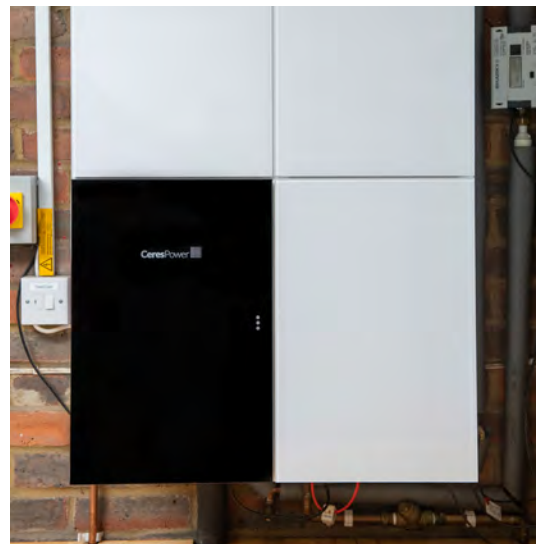
FIGURE 4.1 Sunfire GmbH 2019 Residential SOFC (left) and Ceres Power Ltd 2019 residential SOFC (right)
