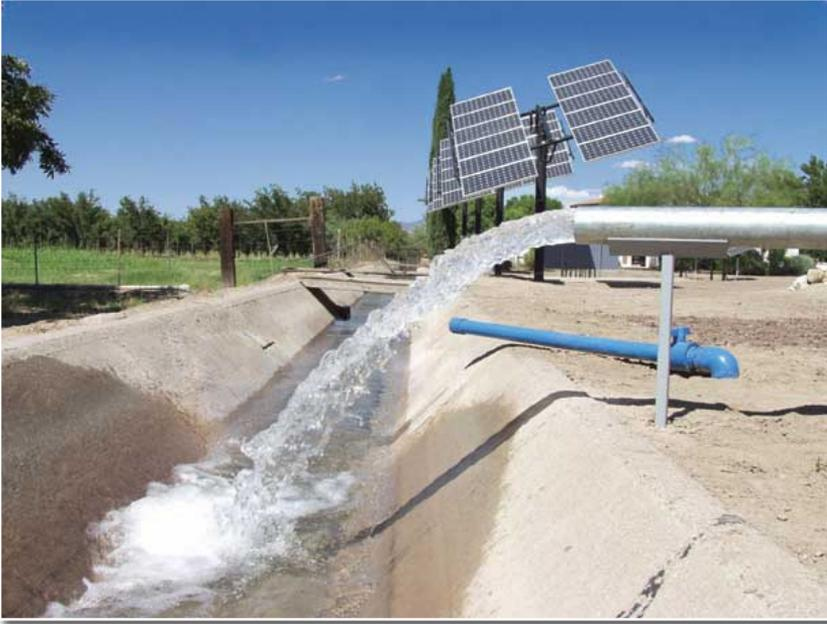
*Water pumping using solar energy*
